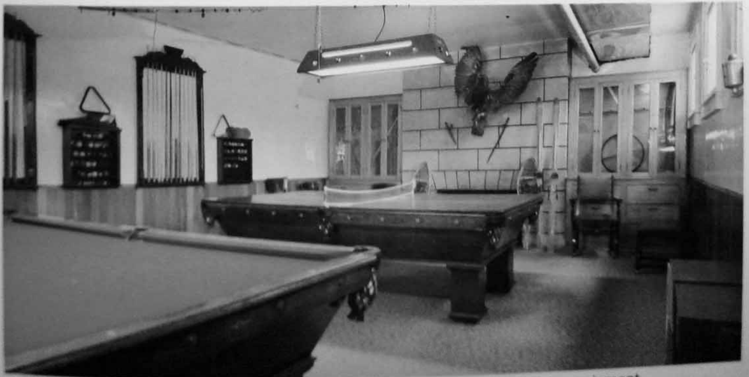
Large indoor recreation has professional sized tables and ample equipment
